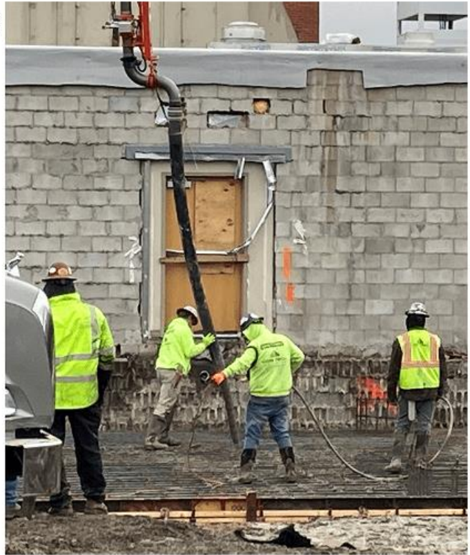
(1) Dump it, (2) pump it, (3) place it. Concrete gets poured. (11-28-22)
