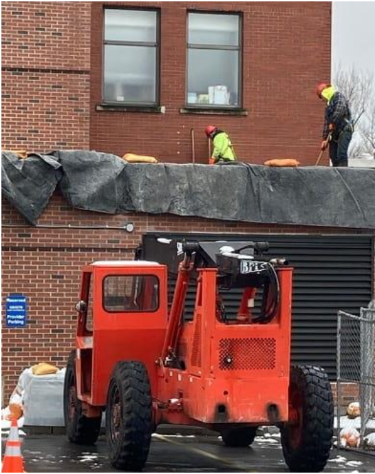
Roofing work is being done in preparation For a new switchgear. (11-16-22)
