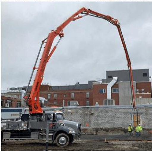
(1) Dump it, (2) pump it, (3) place it. Concrete gets poured. (11-28-22)
