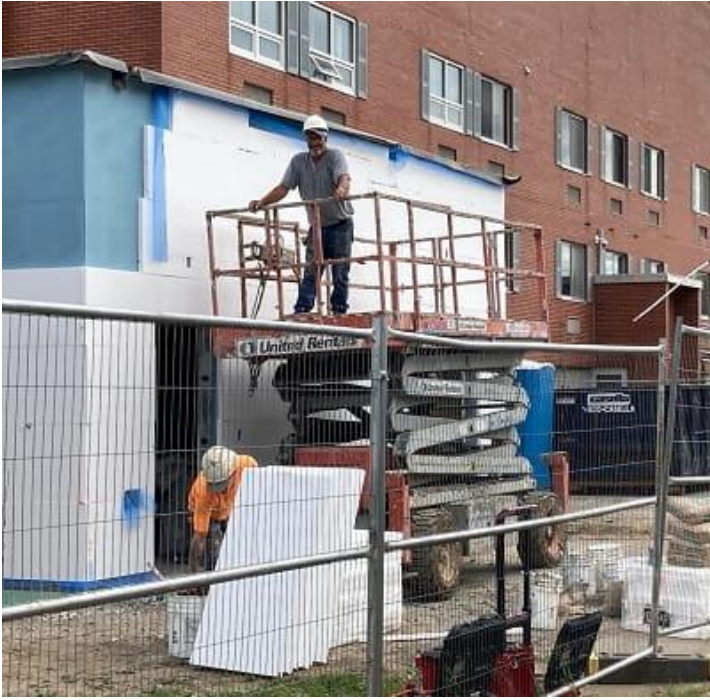
Progress continues on the new Cottage Street entrance to CPH. (9-7-22)
