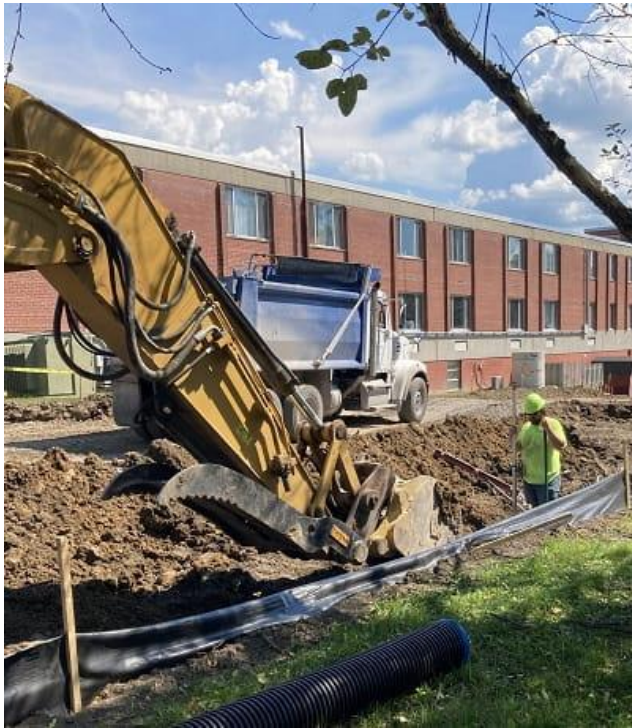
Digging behind CPH's 25 Cottage Street professional building. (8/19/22)
